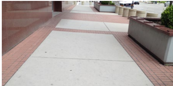
Standard concrete with brick highlights paving pattern
